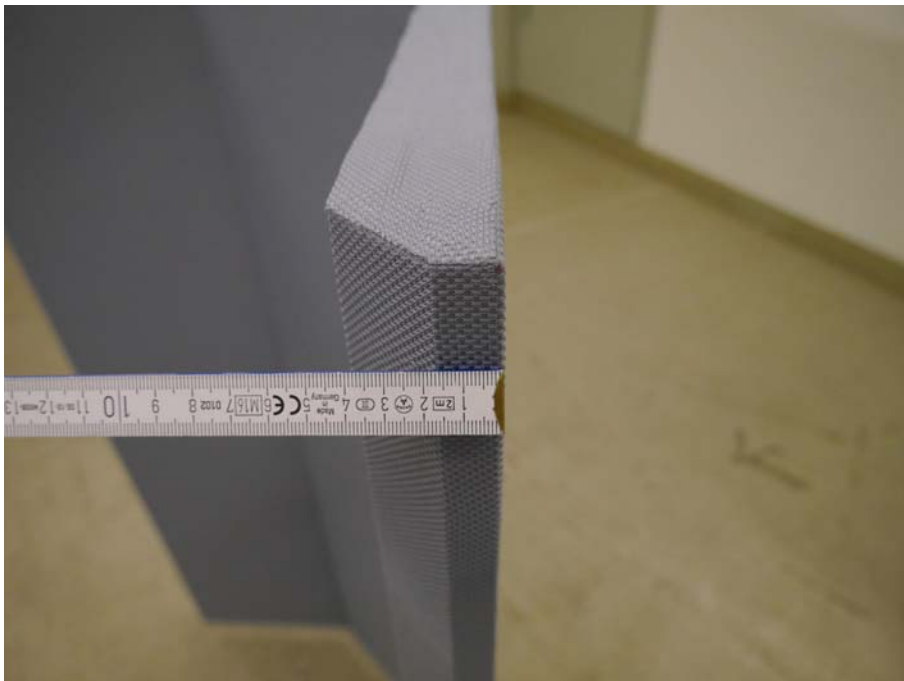
Figure C.2. Execution of the lateral edges.
