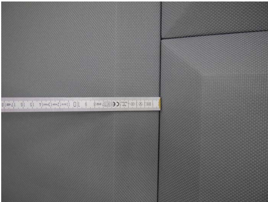
Figure B.2. Wall panels butt-jointed.
