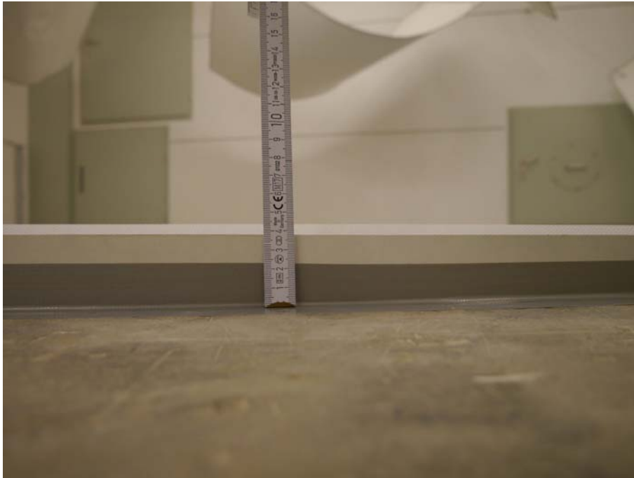
Figure B.3. Circumferential enclosing frame with sealing between frame and floor of the reverberation room.
